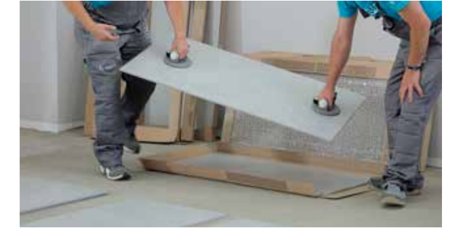
Fig. 7 – Suction clamping elements for large formats
