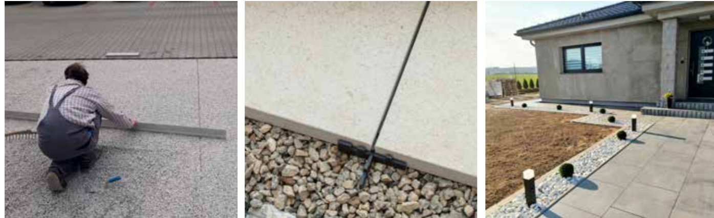
Fig. 28, 29, and 30 – Laying into gravel
