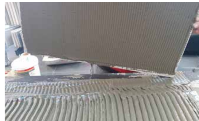
Fig. 10 – Buttering-floating bonding
