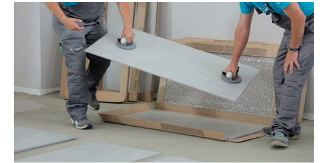
Fig. 7 – Suction clamping elements for large formats
