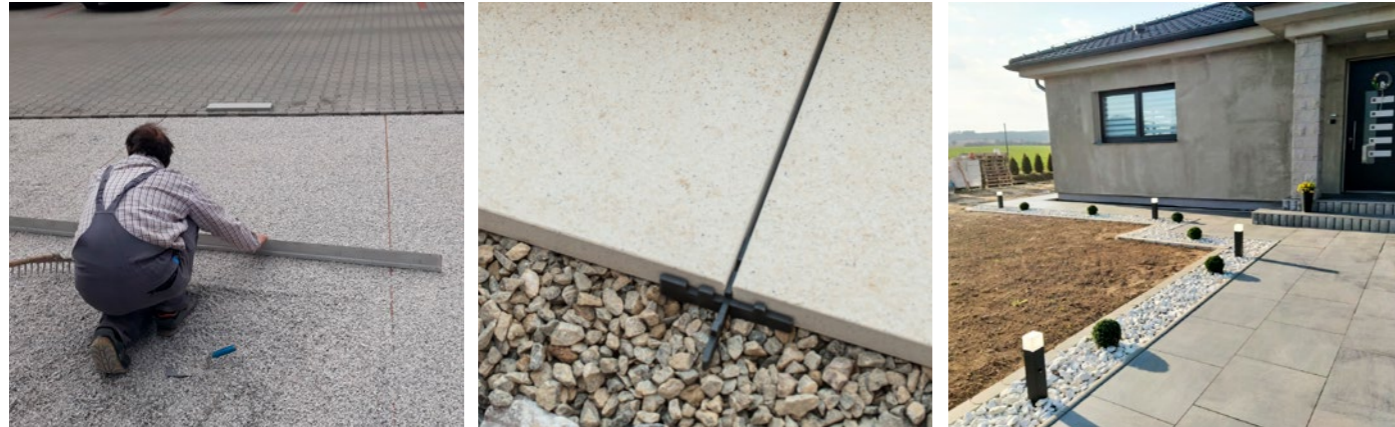
Fig. 28, 29, and 30 – Laying into gravel
