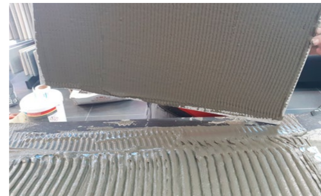
Fig. 10 – Buttering-floating bonding
