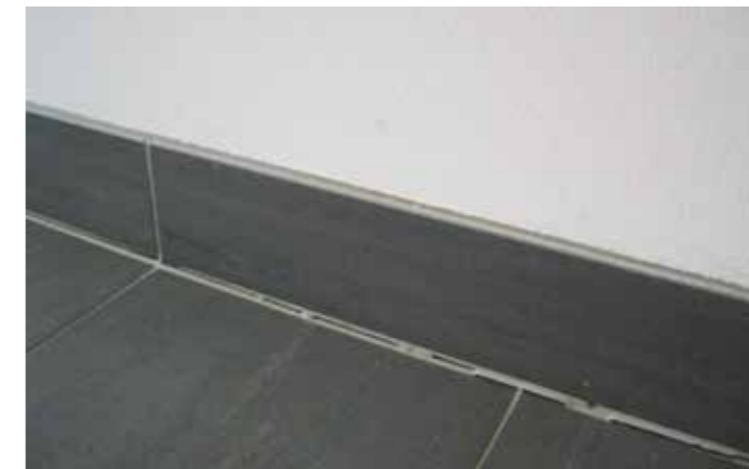
Fig. 26 A cracked expansion joint without the use of a separation cord
