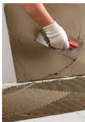
Fig. 13 – Buttering-Floating fixing method
