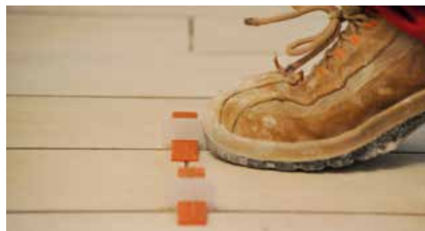
Fig. 9 - Removal of wedges
