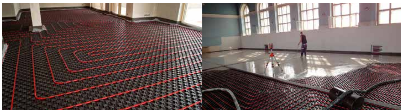
Fig.16 – Example of water-based underfloor heating
