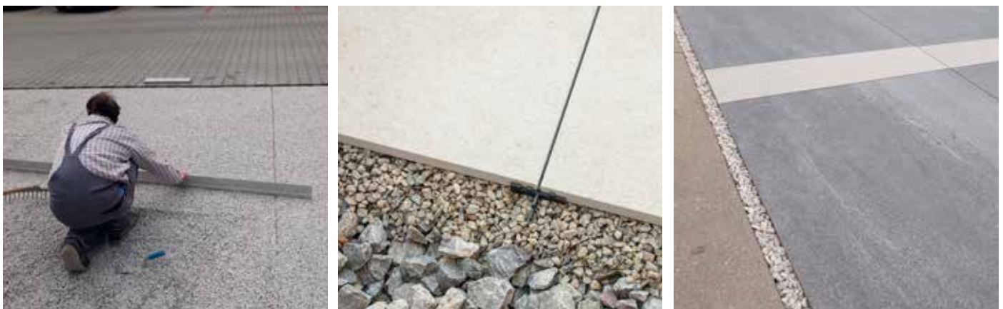
Fig. 22, 23 and 24 - Laying into gravel
