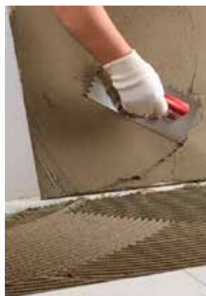
Fig. 13 – Buttering-floating fixing method
