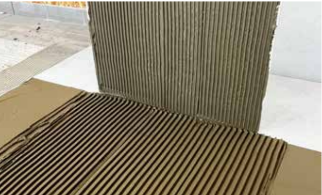
Fig. 10 Buttering-floating bonding
